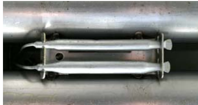
Typical high-limit/sensor probe locations and mounting hardware.
